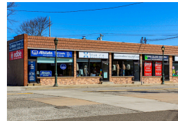
Retail Building North Bellmore, NY
