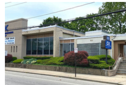
Office Building Hicksville, NY
