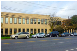
Office Building New Hyde Park, NY
