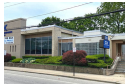
Office Building Hicksville, NY
