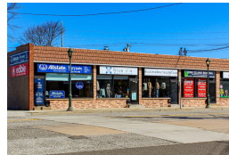
Retail Building North Bellmore, NY
