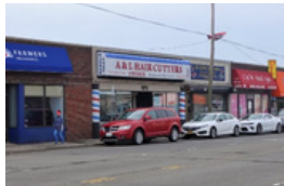
Retail Building Franklin Square, NY
